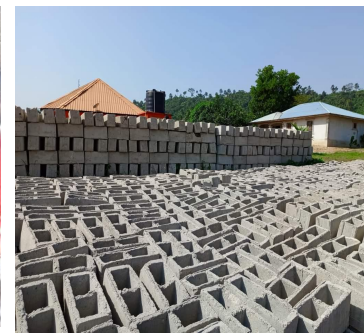
Bricks for Guest House Project
